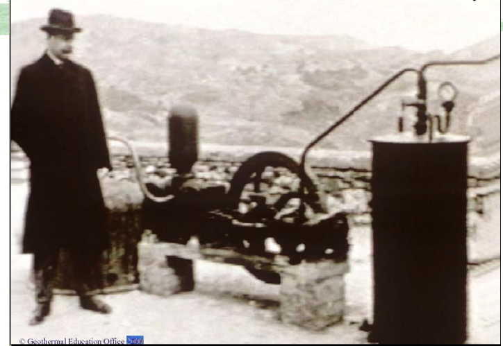
First Geothermal Power Plant, 1904, Larderello, Italy
